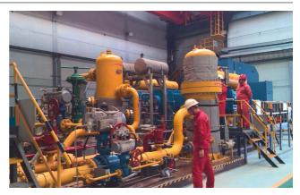
A natural gas storage station used the CRY8129-EX Acoustic Imaging Camera to detect gas pipeline leaks, identifying 8 leak points within one minute.
