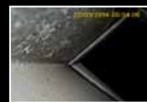
Internal duct work using 28mm detachable camera head (VSC28)
