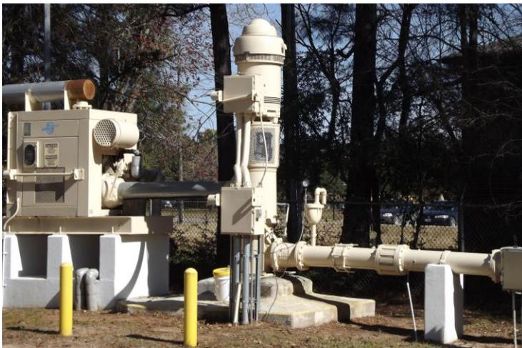
*Deep well vertical pump and 400 HP motor at Well-1 Pumping Facility*
